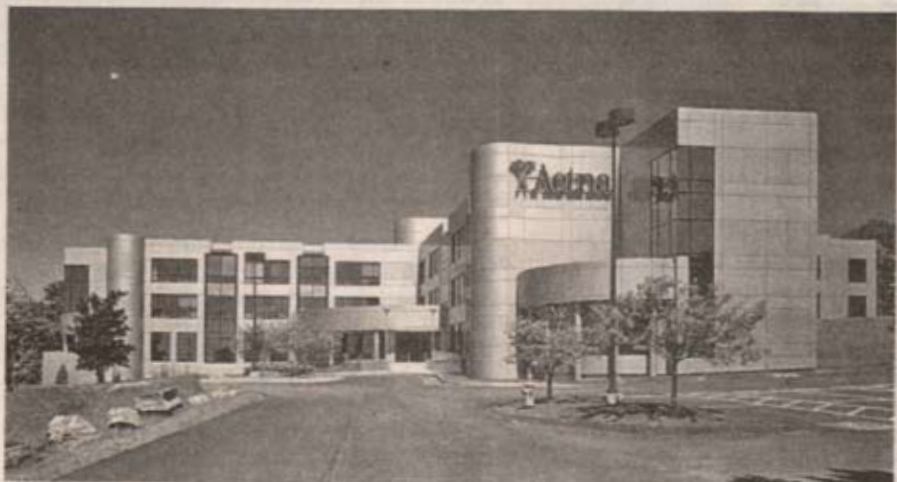
Dead River Properties has transformed the former Spring Harbor psychiatric hospital into high-end office space .
